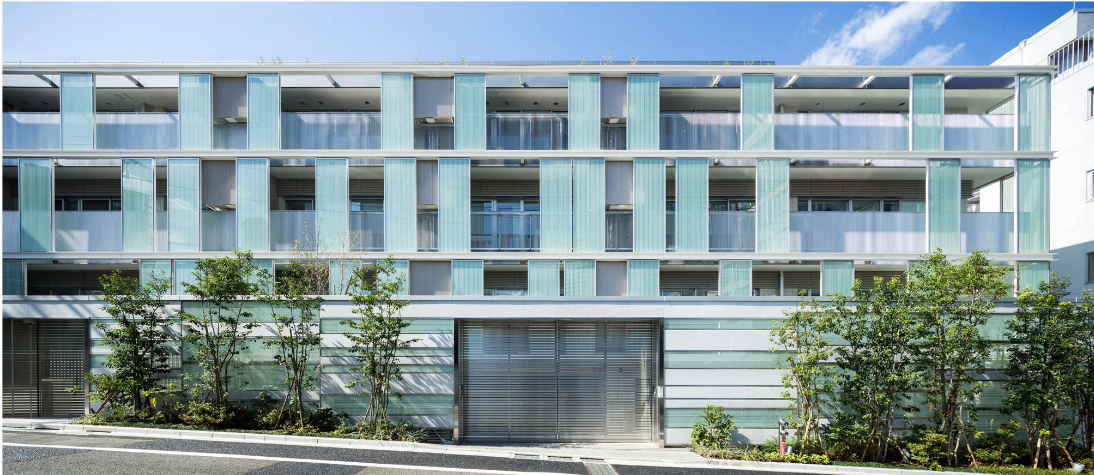
Stacked layers of materials such as printed glass screen, stone, metal, lattice handrail, etc., it is to form a multi-layered facade
