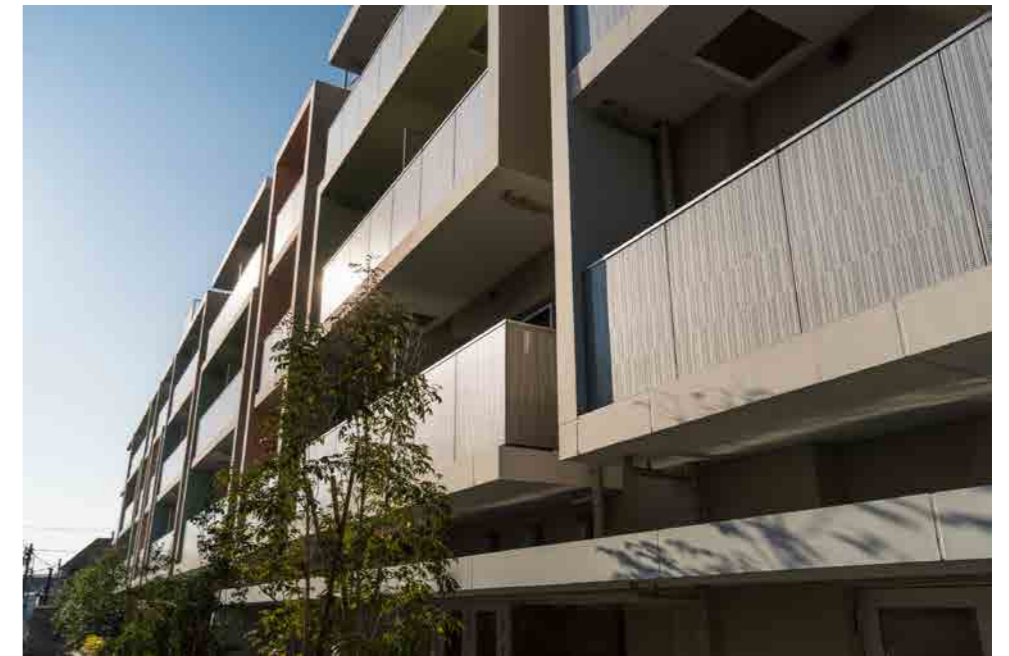
Handrails with aluminum punched panels with the image of Kasuri pattern.
