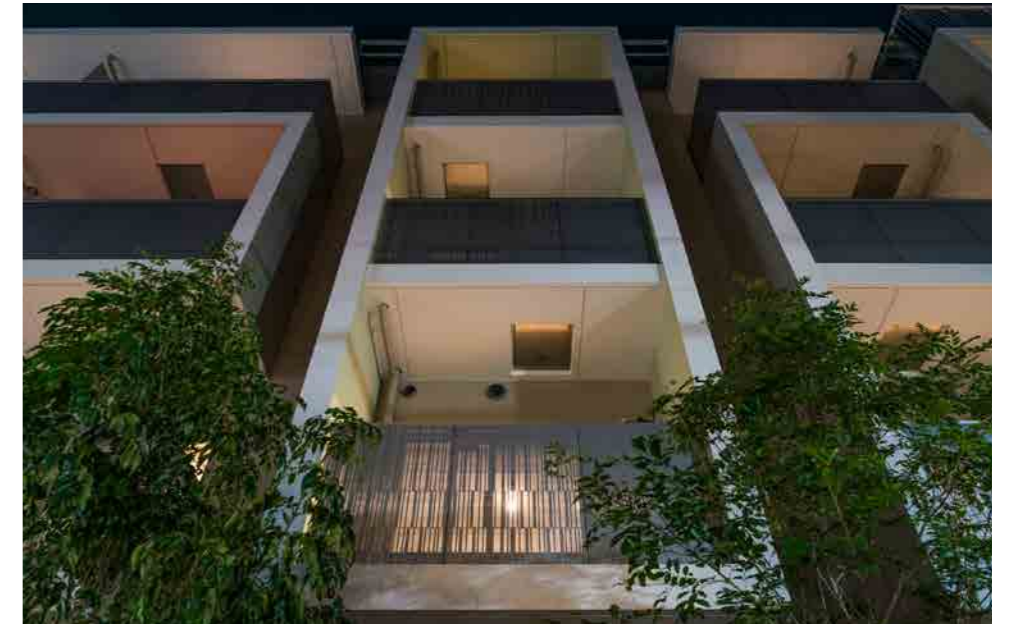
Five colors are applied on the inner wall of the balcony that is enclosed by square shape.
