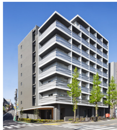
Intersection facing open-terrace and entrance
