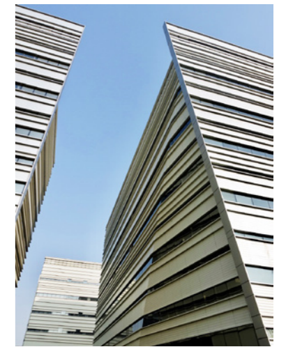
Looking up at the main gate. One side wall is slanted due to the reason of making it shapes as the character "ba (8)" that requested by Fengshui
